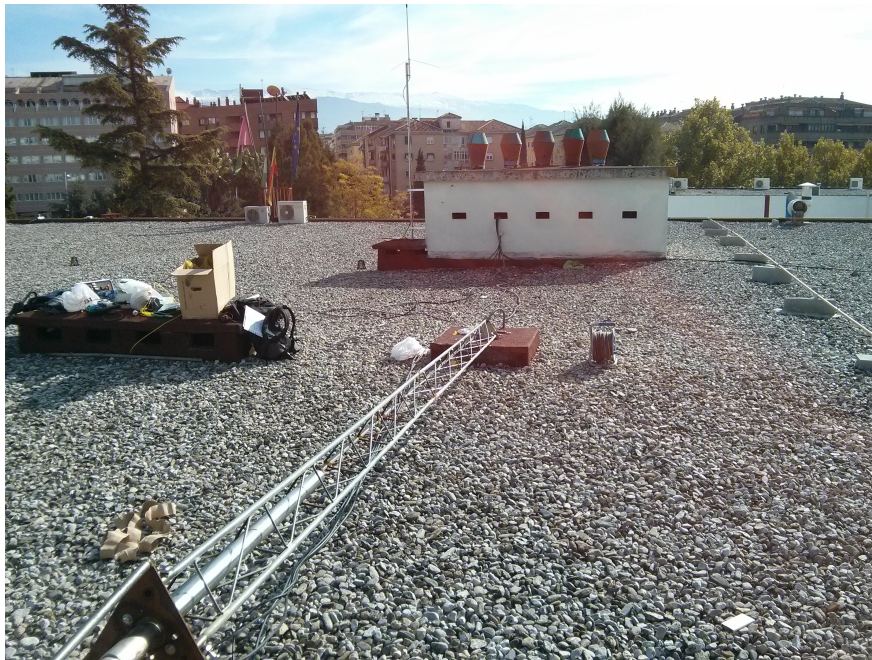
Figure 6.3 – Mast of the X-Quad antennas
