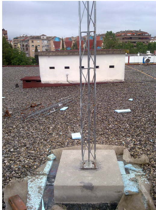
Figure 6.1 – Base of the mast
