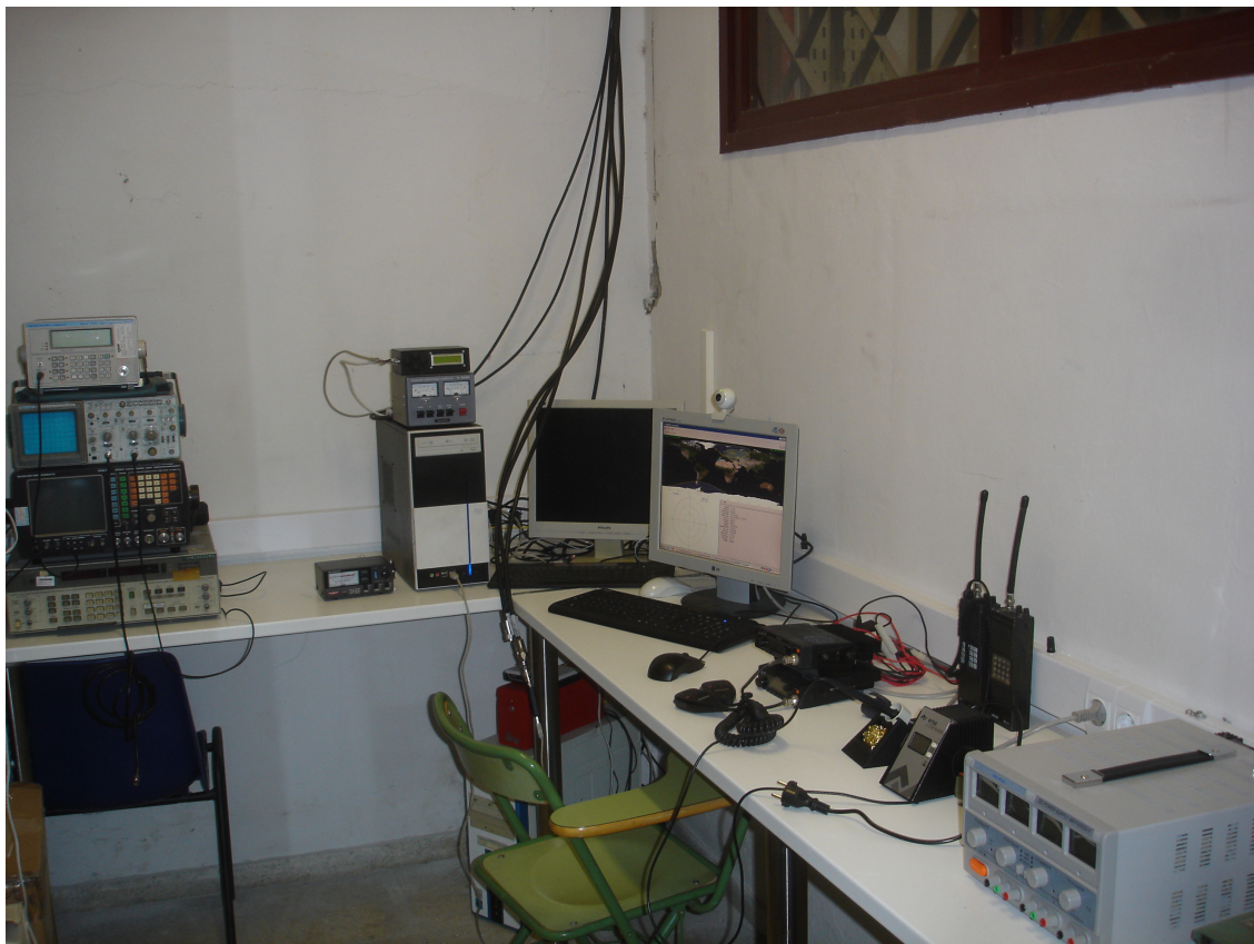
Figure 6.18 – Equipment on the control room
