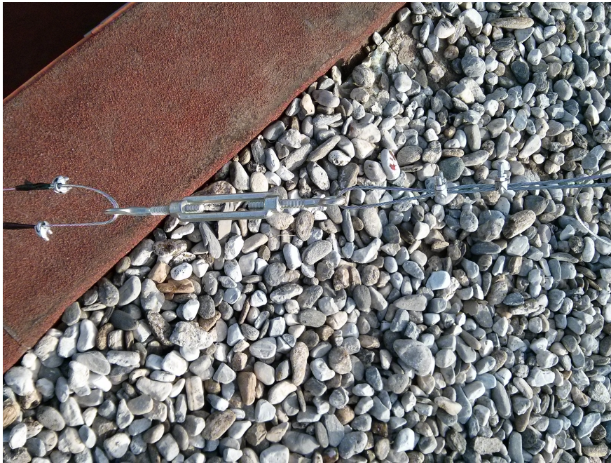
Figure 6.4 – Attachment of the cords to the floor
