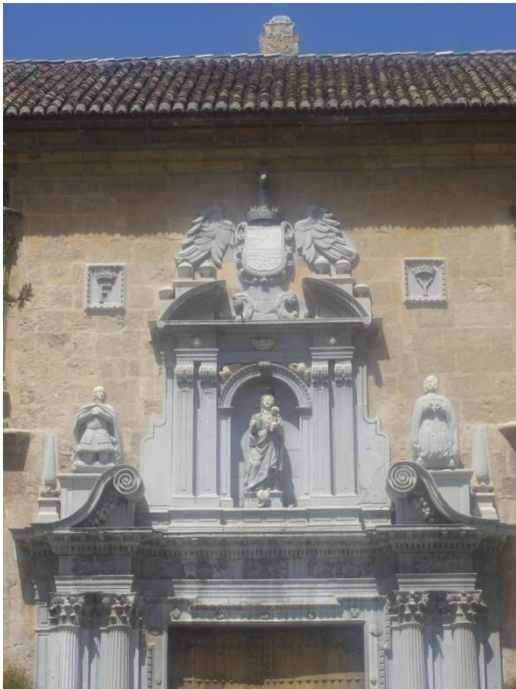
Fachada Hospital Real
