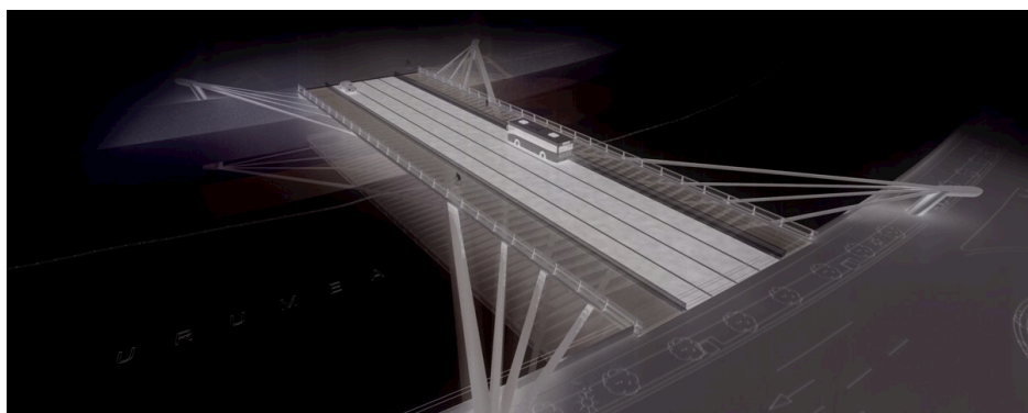
Figure 9.1: Example of a novel infrastructural application involving an all-composite bridge made of carbon and glass fiber-reinforced polymers. 2
