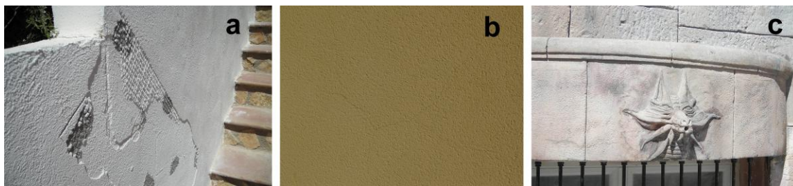
Figure 4 Example of render application on a polyester mesh (a) and renders with trowelled (b) and sculpted (c) finishes.
