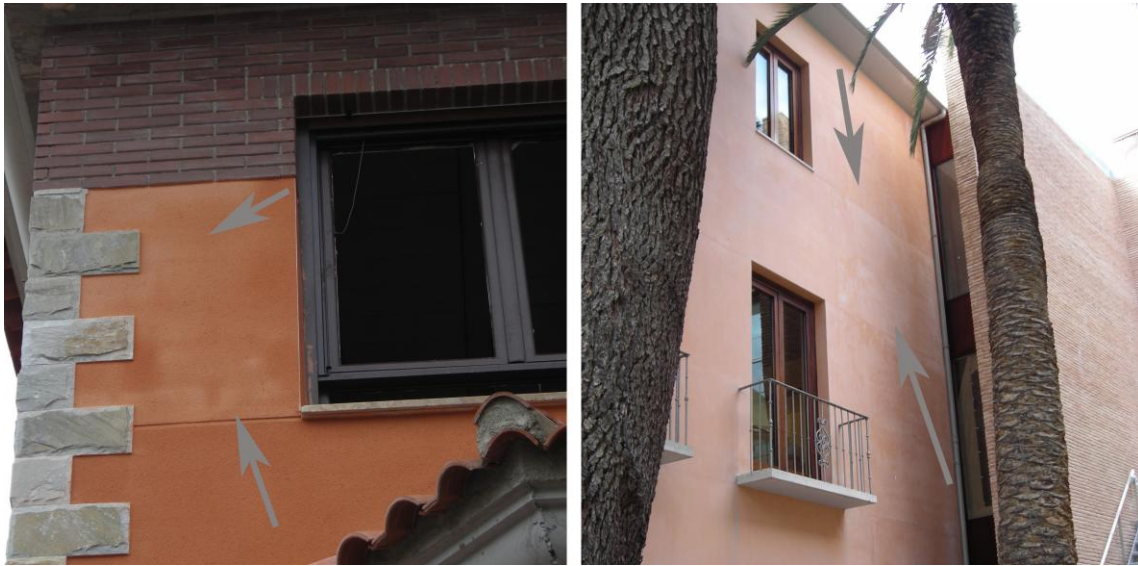
Figure 3 Examples of bad rendering: the second layer has been applied before the first one was completely dry and this has produced large, irregular spots that alter the final colour.
