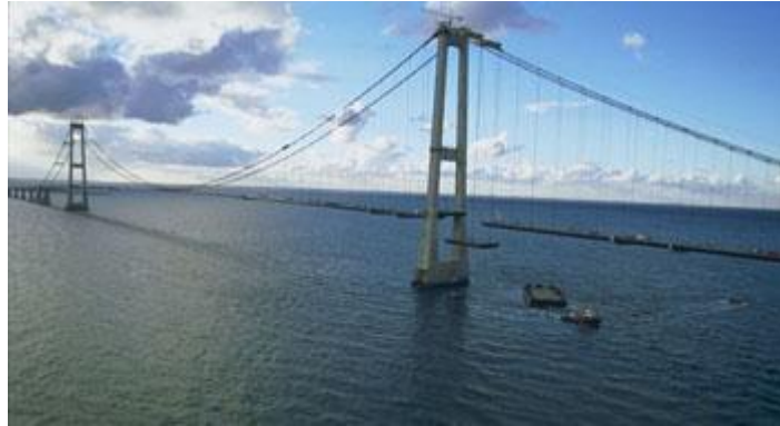
Figure [A1- 2]: View of the Storebælt's main span under construction [75].
