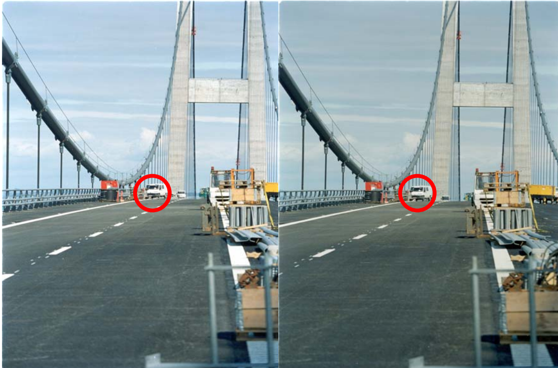
Figure [1- 1]: Vertical vortex induced oscillations observed in the Storebælt East Bridge [17]. May 1998. The marked vehicle is stationary. The location of the camera is the same for both images.
