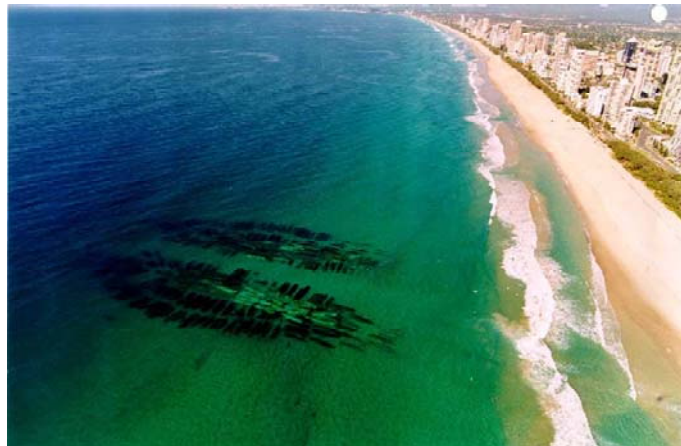
Fig. 1. Aerial view of the Artificial Surf Break at the Gold Coast, Australia. The structure is V-shaped in plan with the apex pointing seaward (courtesy of International Coastal Management, Australia, www.coastalmanagement.com.au ).
