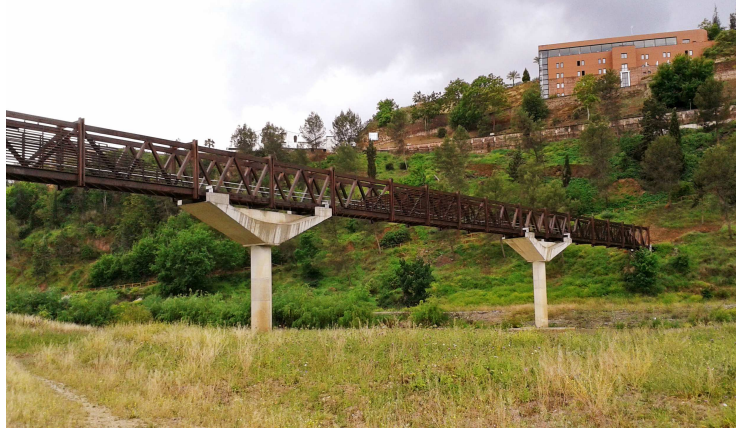
(a) Montoro bridge over the Guadalquivir river
