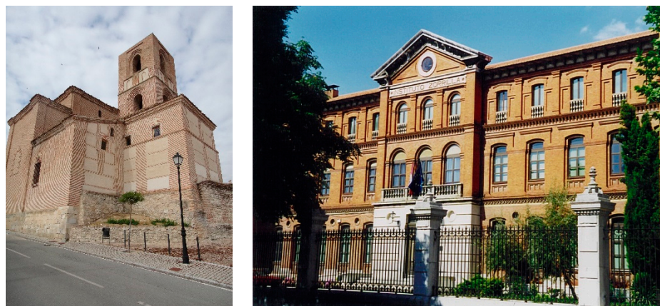
Figure 1. On the left, Mudejar church of Arévalo, Ávila (handmade bricks), and on the right, Institute Zorrilla, Valladolid (mechanical bricks).
