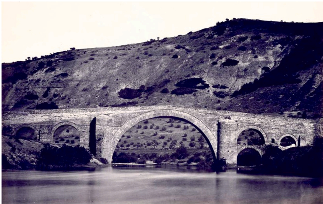
Fig. 2. View of the Ariza Bridge in the mid-19th century.
