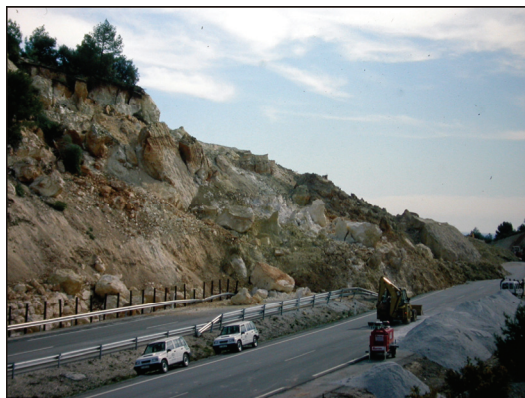
Figure 8-2. Panoramic view of the toe of the Diezma landslide during the 2001 collapse over the A-92 motorway, which was closed for several days.
