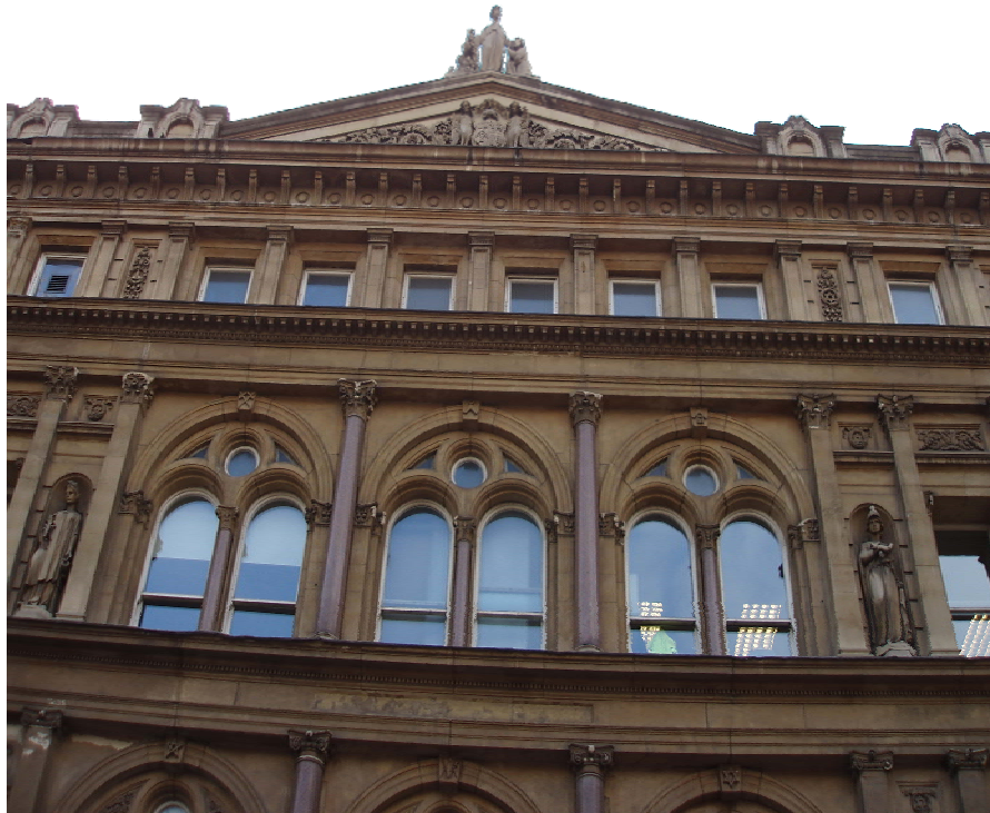
Freemasons Hall, Cooper Street. Manchester. William Mangnall, 1863.
