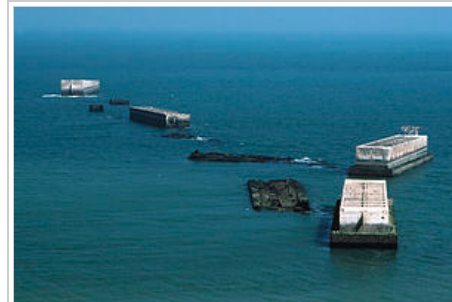
A line of Phoenix elements forming a breakwater at Arromanches
