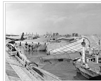
Wrecked pontoon causeway of one of the "Mulberry" artificial harbours, following the storm of 19–22 June 1944.
