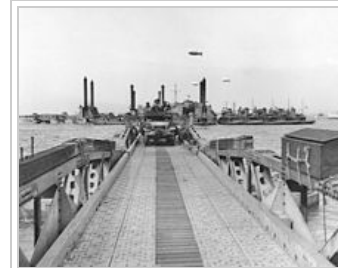
A Whale floating roadway leading to a Spud pier at Mulberry A off Omaha Beach
