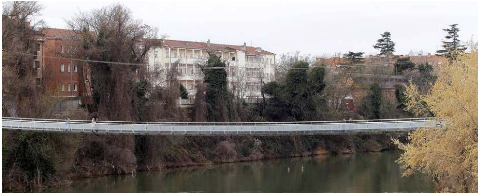
Figure 1. Pedro Gómez Bosque footbridge. Landscape view.
