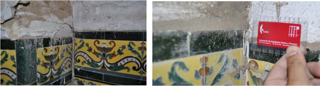
Figures 2 y 3. Offset between tiled baseboards.
