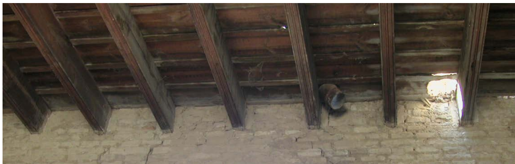
Figure 9. Floor constructed with wooden beams and planking.
