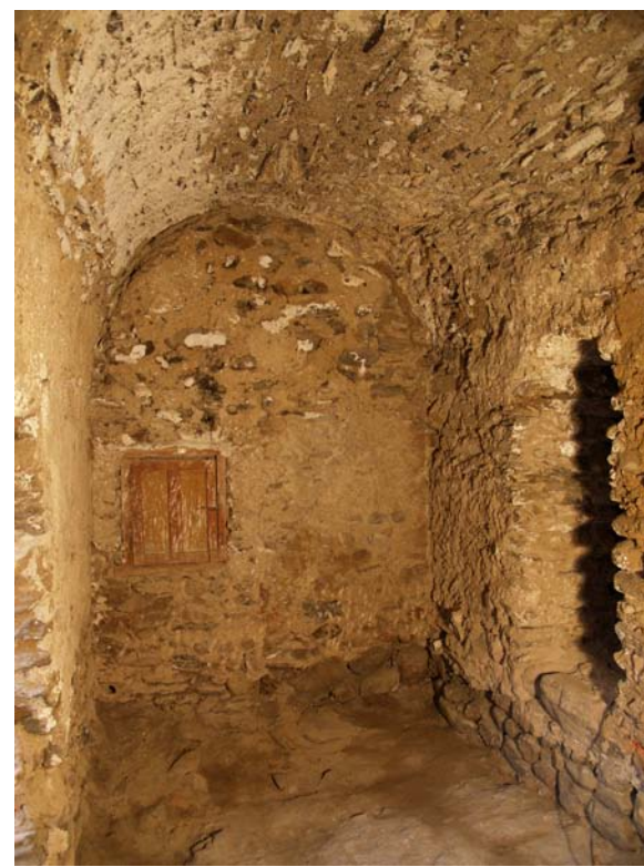
Sala 1 (frigidarium), vista norte. [393]
