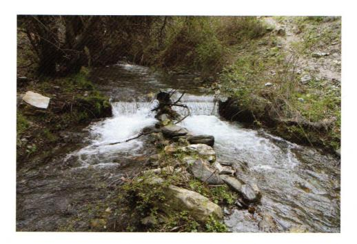
Fig. 7. Dam for the Alhama river system in the same place where the XIIth century's document mentioned the *Maqsam* to distribute the water into the two main channels.
