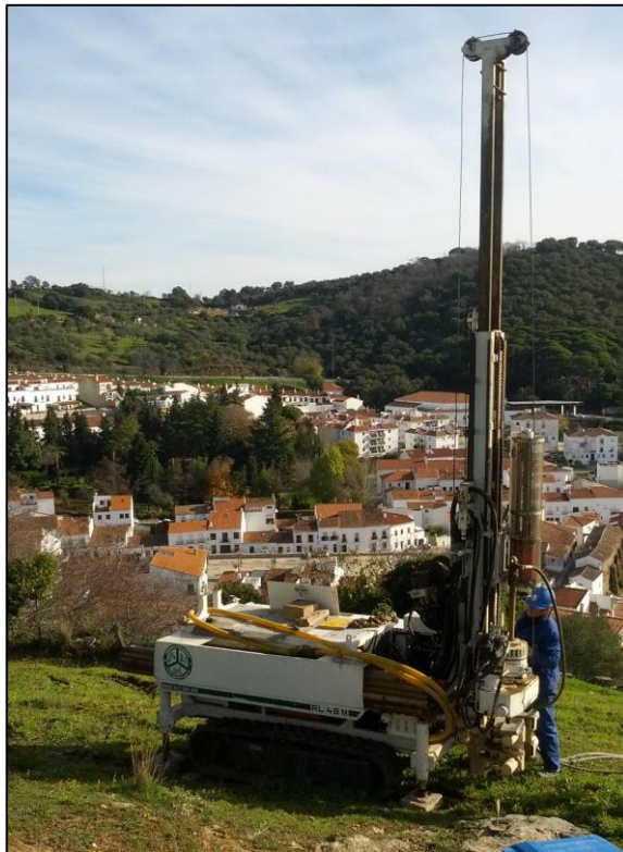
Figure 8.1: Rolatec RL 48-M equipment on the borehole 1.
