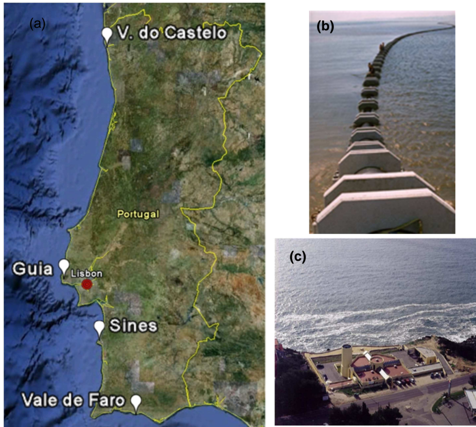
Figure 3-4 (a) Submarine outfall location for the case studies; (b) Treatment plant of Guia, Cascais; (c) Submarine outfall of Guia.
