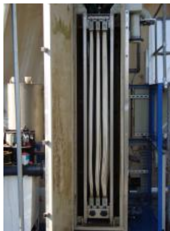
Figure 3.8. Interior view of the MBR in the UF plant.
