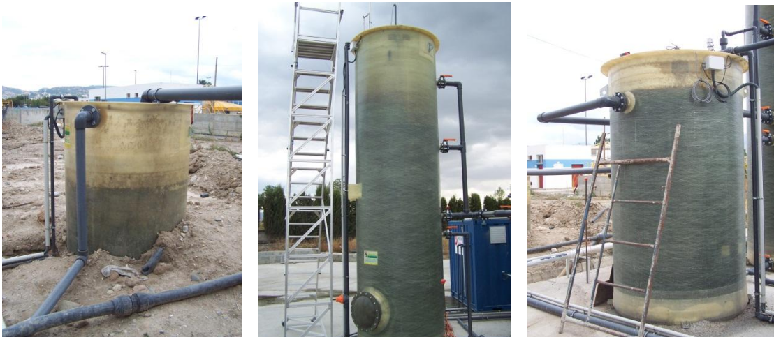
Figure 3.2. Anoxic bioreactor (left), aerobic bioreactor (center) and MBR (right) in the MF plant.
